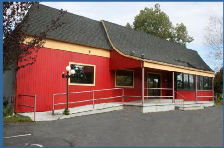
9,480 SF vacant restaurant on subject property
