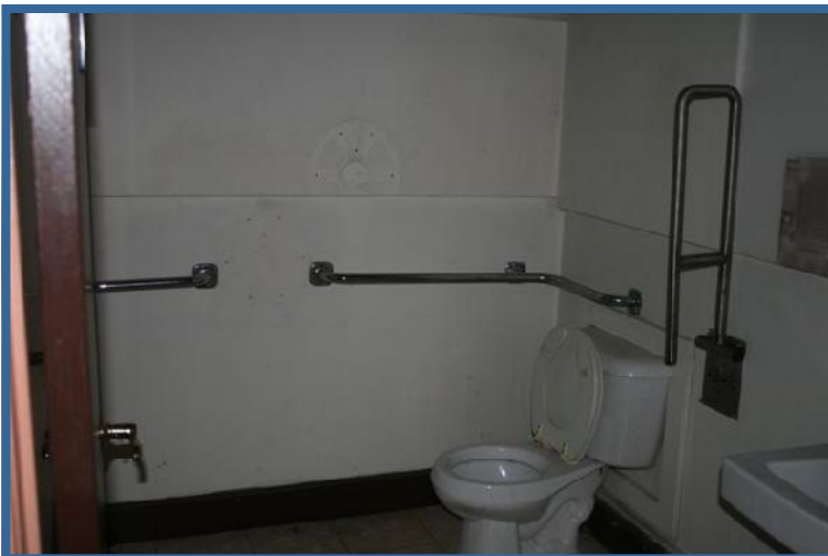
Handicap Accessible Restrooms
